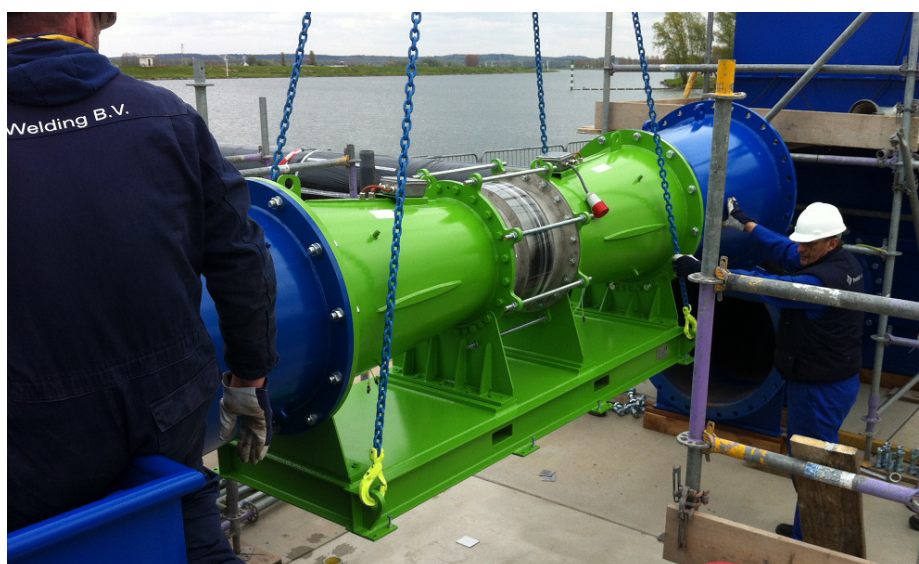
Figure 2.4 Lifting the modified bulb turbine (venturi-type) into position into Pro-Tide's field-laboratory, for tests on fish friendliness, Maurik, May 2015.
